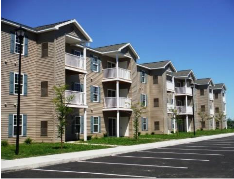
Figure B. Parking area without accessible parking or curb cuts, online photo from apartments.com of Camillus Pointe Senior Apartments, Camillus, New York.
