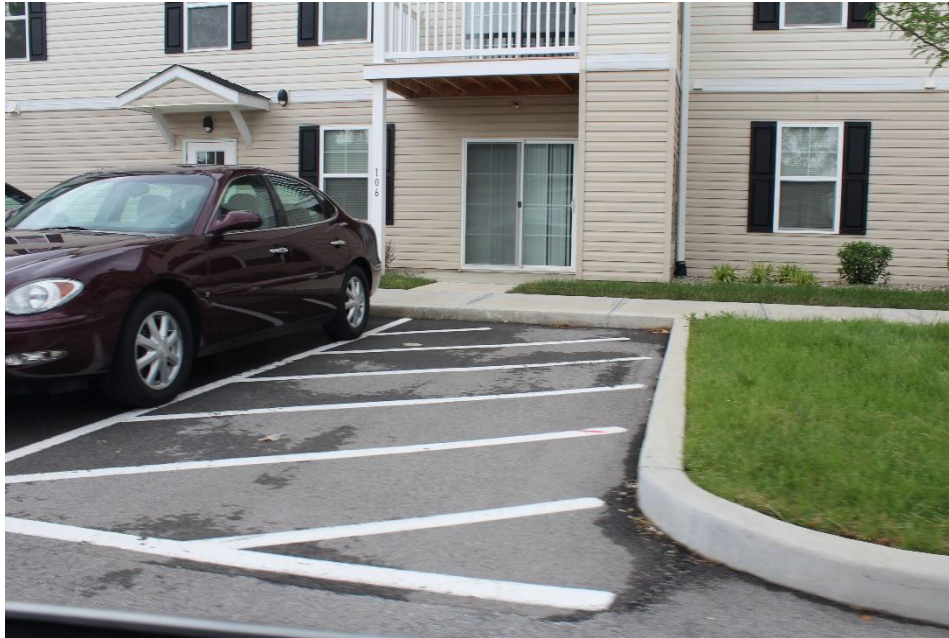
Figure D. Striped access area without curb cut at Pleasant Run Senior Apartments, Indianapolis, Indiana.
