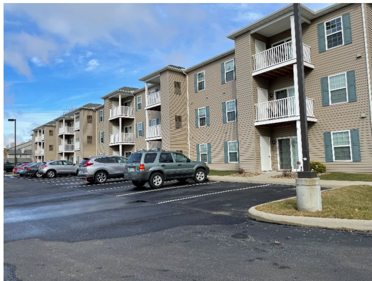
Figure A. Parking area without accessible parking or curb cuts at Parma Village Senior Apartments, Parma, Ohio.
