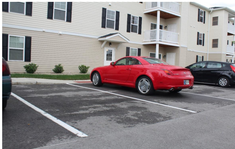
Figure C. Car blocking curb cut with no access aisle at Pleasant Run Senior Apartments, Indianapolis, Indiana.
